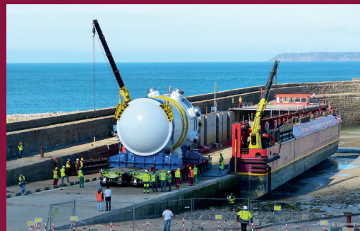
485te Reactor offloaded at Dielette en route to Flamanville Nuclear Power Station
