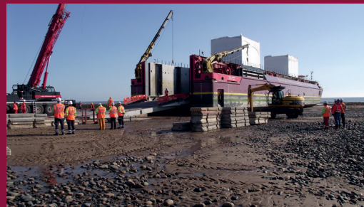
2 of 11 modules. Heaviest of which was 565te. Sellafield, Cumbria.
