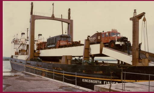
Kingsnorth Fisher offloads at Combswich Wharf April 1972
